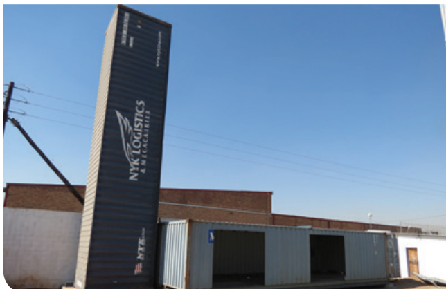
The construction of the Mabopane Local Enterprise Centre.
